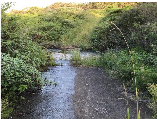
Concrete culvert at Ck crossing (CP 5)
