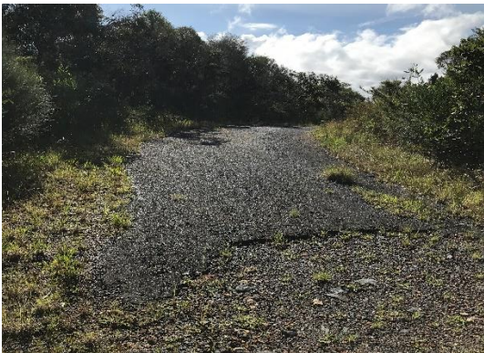
Start of the tarmac road (CP 2)
