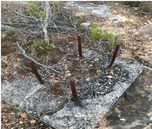
Danger – Steel Spikes at Quarry
