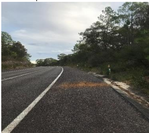
Parking on Pacific Highway verge
