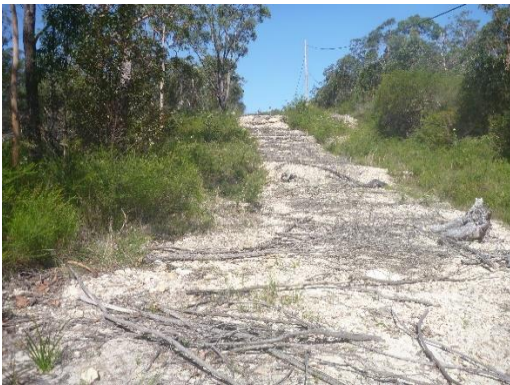
At CP 6 looking back up the "Steps"
