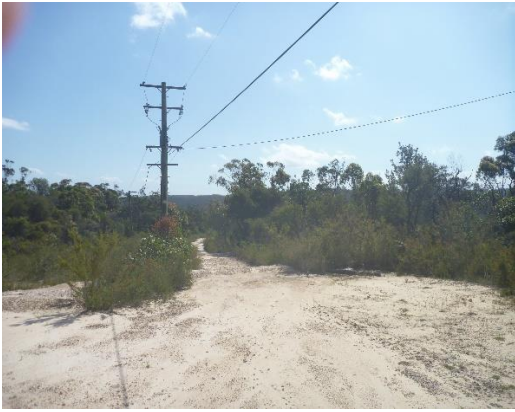
TK under the powerlines to the WSW
