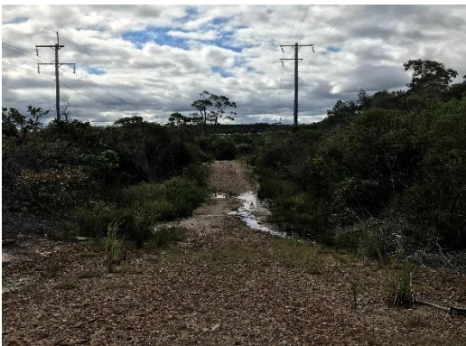
Creek crossing & power posts (CP 4)
