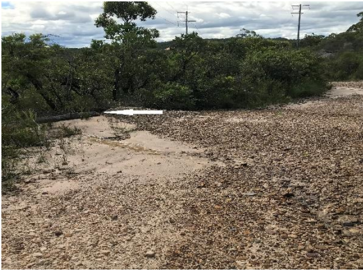
The erosion control cutting (CP 3)
