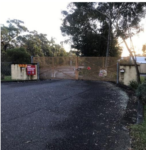
The Kariong Fire Centre
